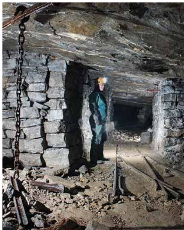
A roadway with mid-20th century tramway points, running between late 19th century waste packs in Holme Bank Chert Mine (Copyright: Mat and Niki Adlam Stiles).
