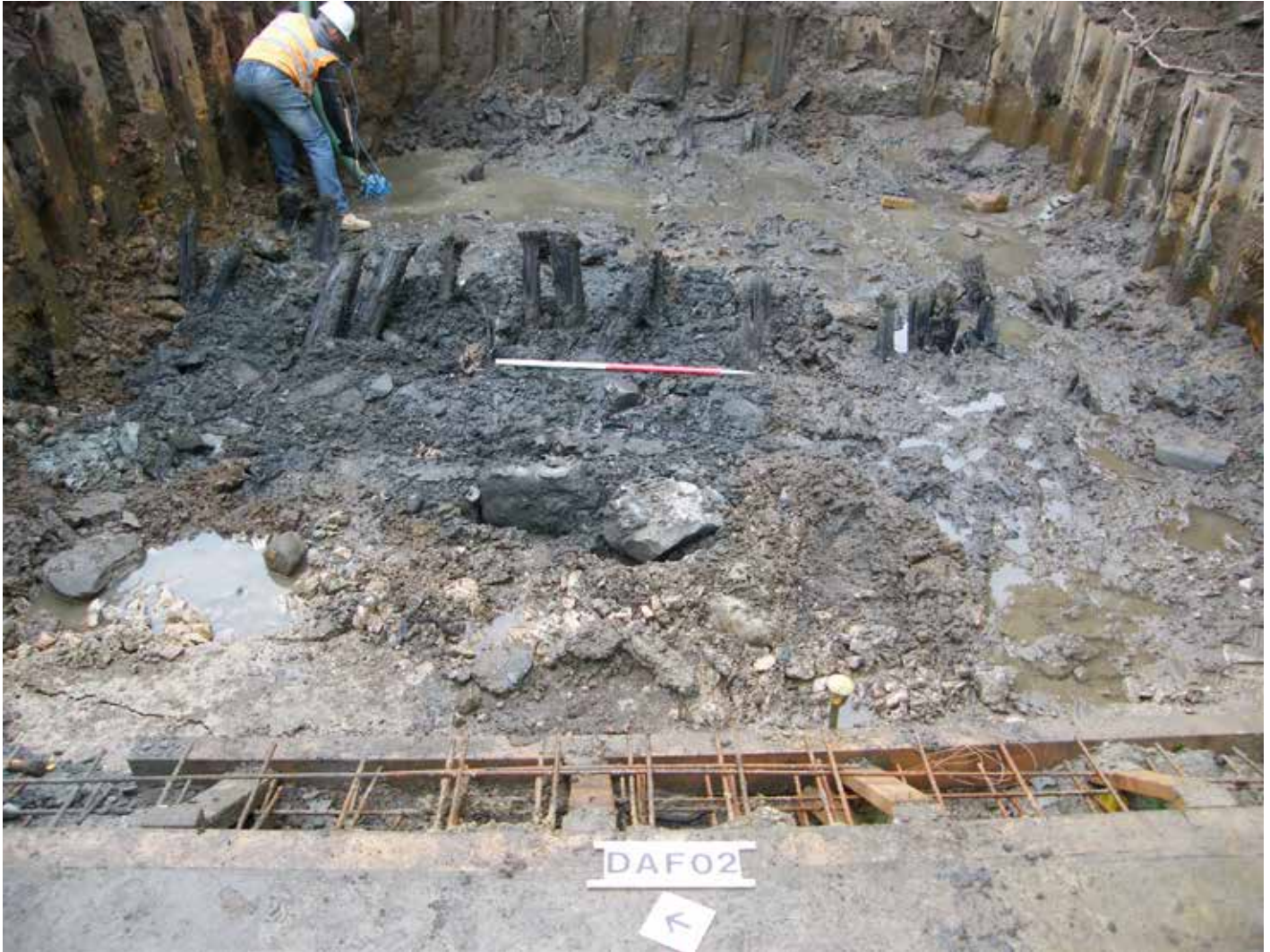
The westernmost wall and row of timbers
