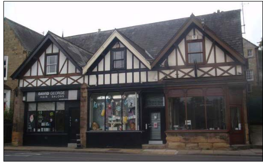
P5.57 Vernacular Revival building on Buxton Road
