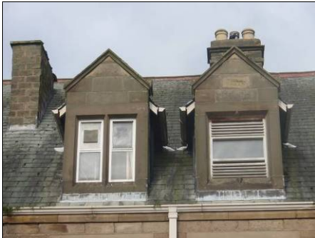
P5.60 Gabled dormers which are wholly in the roof-space
