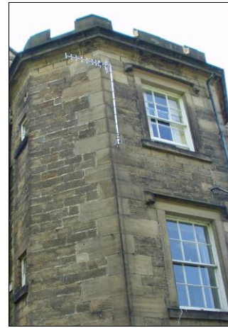
P5.35 Bridge House exhibits both classical and gothic detailing
