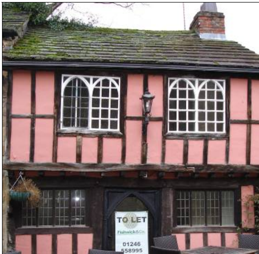
P5.8 This timber-framed building in Avenel Court was constructed in the twentieth century
