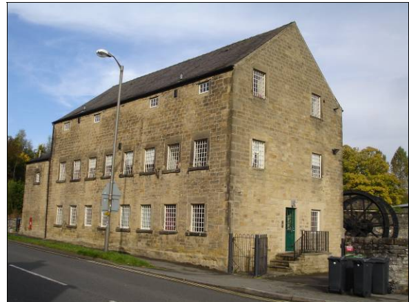
P5.49 Victoria Mill, Buxton Road
