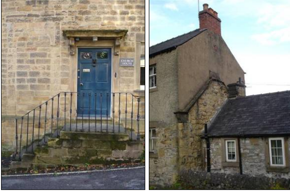
P5.7 Left: Evidence of blocked door next to existing entrance. Right: The remains of an earlier building, on a gable end
