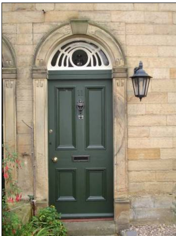
P5.30 Nineteenth century door detail on South Church Street
