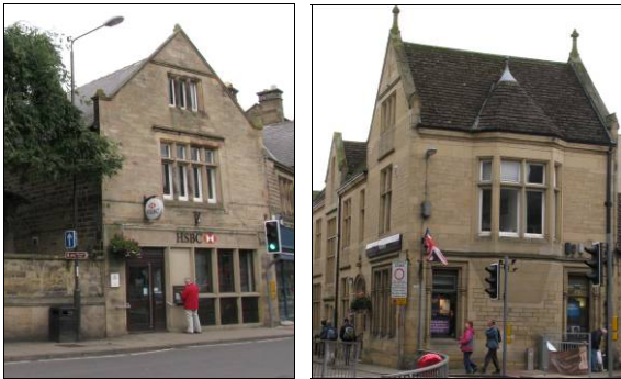
P5.42 HSBC, left, and Nat West Bank, right are nineteenth century buildings which have Gothic details
