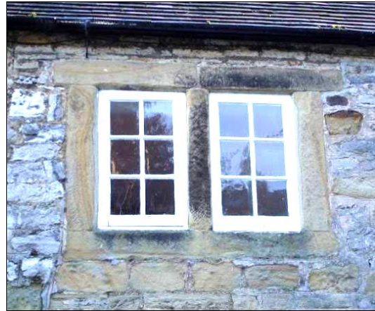
P5.21 Eighteenth century window surrounds square cut, with oversailing lintels
