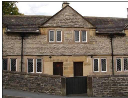
P5.18 St John's Almshouses have seventeenth century details but arranged in an eighteenth century symmetrical layout
