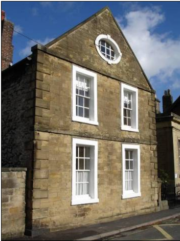
P5.19 Bank House oeil-de-boeuf window
