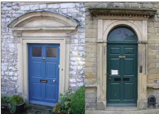
P5.20 Pedimented door surrounds with fine moulded detailing
