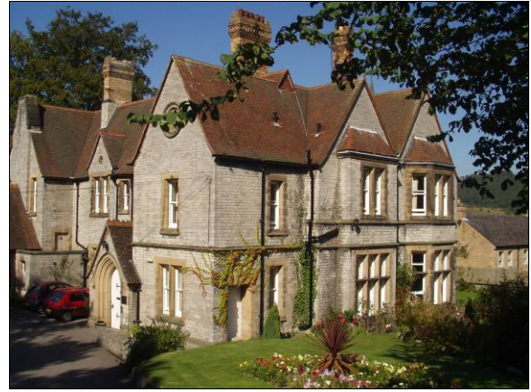
P5.43 Edward Balston's Vicarage by Alfred Waterhouse
