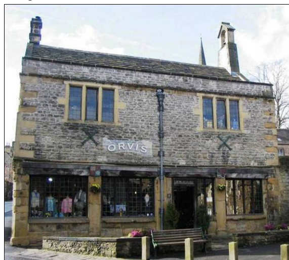
P5.14 The Old Town Hall, the ground floor arcade has been in-filled with shop windows
