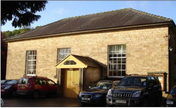
P5.45 The Friends' Meeting House off Matlock Street above, and The Wesleyan Reform Chapel, Little Bagshaw Hill, below, are Churches in the Classical style
