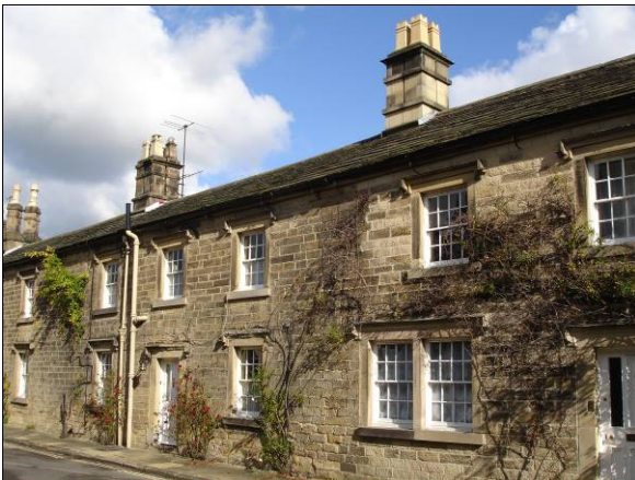
P5.34 Castle Street, the hoodmoulds over the windows reflect Gothic architecture
