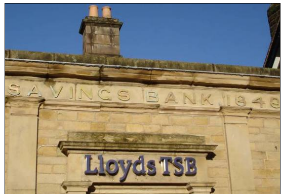
P5.40 Classically detailed pediment and pilasters at the Lloyds TSB Bank
