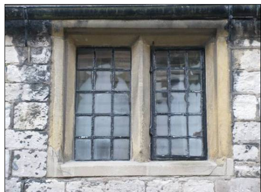
P5.10 Typical seventeenth century window, with double chamfered surround
