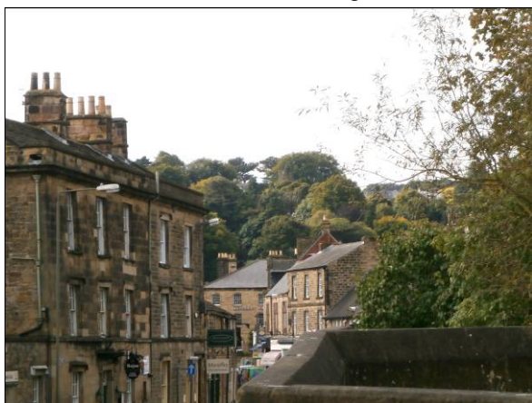
P5.1 The density of the buildings is high in the town centre
