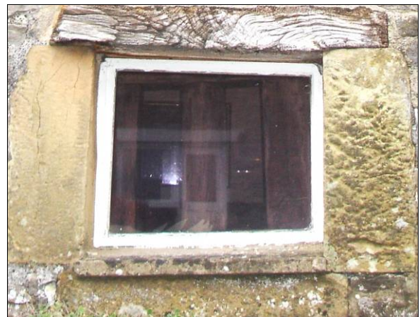
P5.6 Sixteenth century wooden mullion window at the Old House Museum (behind a modern glazed window)
