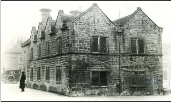
P5.15 The outline of the arcade arches can be seen on the ground floor of the gable end
