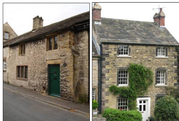
P5.3 Left, a seventeenth century vernacular cottage. Right, a nineteenth century house with symmetrical, polite detailing
