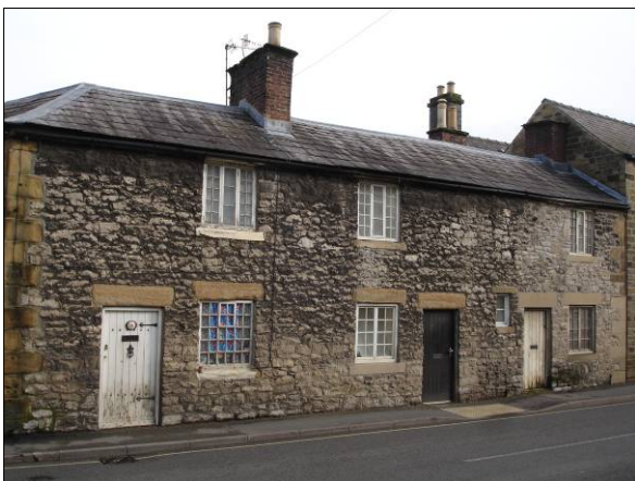
P5.23 Arkwright Cottages on Buxton Road, note at the left of the row, the quoins to the end of the wall and the ground floor metal window
