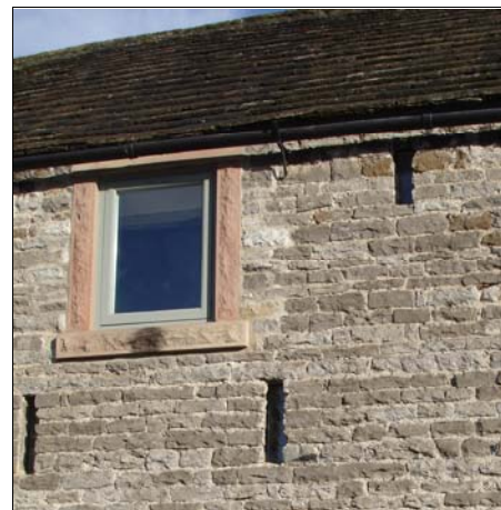
P5.64 The ventilation slots, now glazed, indicate a previous agricultural use
