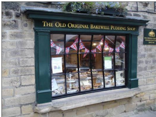
P5.52 An early nineteenth century shop window
