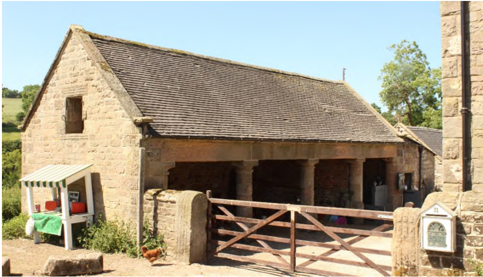
Figure 3.7 An open-fronted cartshed located adjacent to the entrance to the farmstead
