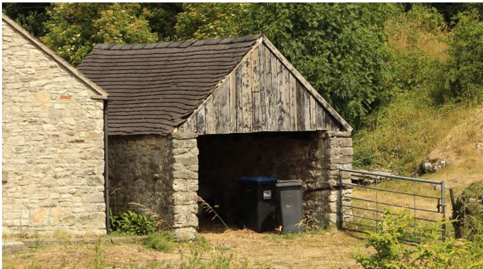
Figure 3.8 A cartshed with an open gable end
