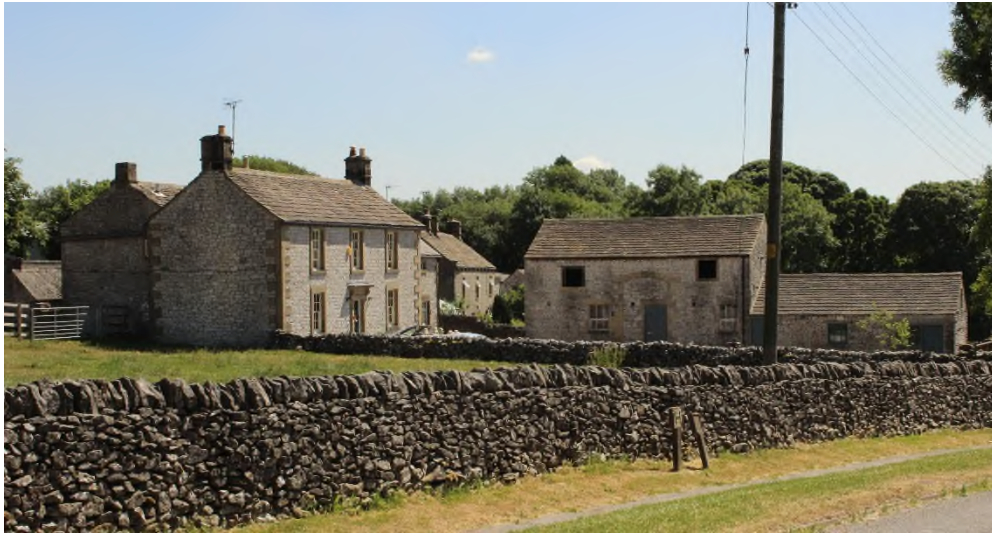
Figure 3.15 A loose courtyard with a building range to one side. The two storey building was constructed as a combination barn, the threshing bay being later blocked and the building turned to serve solely as animal housing and hay storage.
