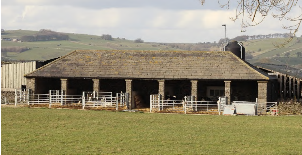
Figure 3.5 Open-fronted shelter sheds are typically associated with mid- to late 19 th century courtyard farmsteads built by estates.
