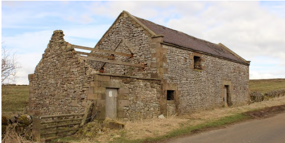
Figure 3.20 an 18 th century field barn. The main body of the building is divided into two parts, one part aisled to the rear (see Figure 3.21).
