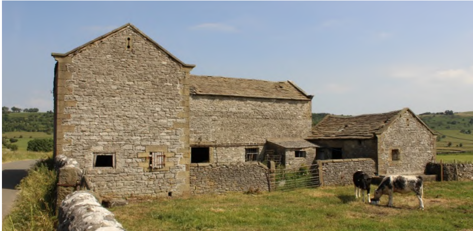
Figure 3.18 An example of a large outfarm group with a cattle yard. Examination of the masonry of the central range shows that there are several phases of construction and remains of an earlier field barn may be incorporated into the group – there is often more than one phase of construction in these isolated buildings suggesting changing requirements over time.
