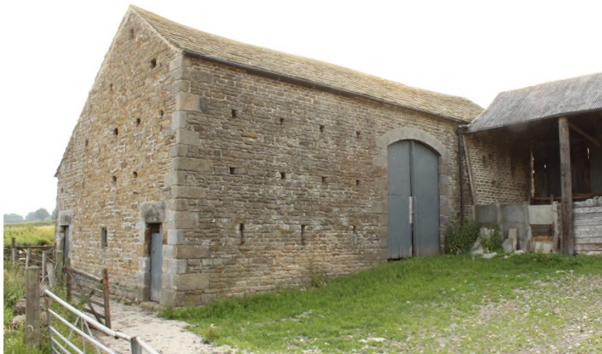
Figure 3.2 A combination barn with cattle housing at the lower, left hand end and the threshing bay and hay and crop storage to the right and above the cattle.
