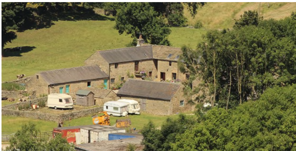
Figure 3.12 A L-plan (house attached) group. As with many linear and L-plan farmsteads, there are other smaller detached buildings within the group.
