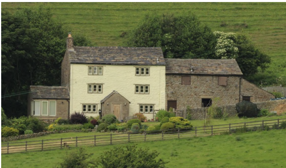
Figure 3.11 A medium-sized linear range with house and working buildings clearly of different phases.
