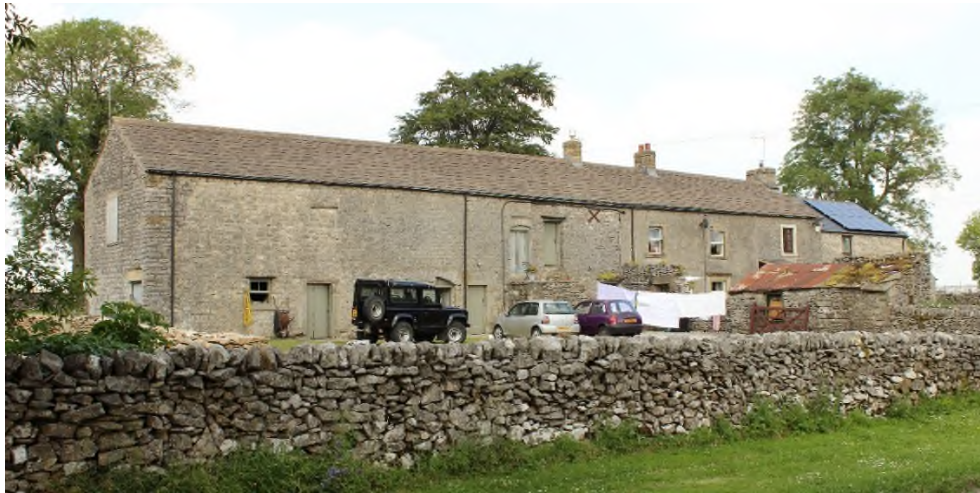
Figure 3.10 A large linear range with a continuous roofline across house and working buildings.
