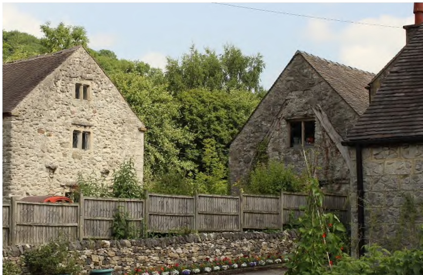
Figure 3.1 The gable of the barn to the centre of the photograph shows the remains of a cruck truss, probably of an earlier barn fossilised within the wall of the enlarged building.
