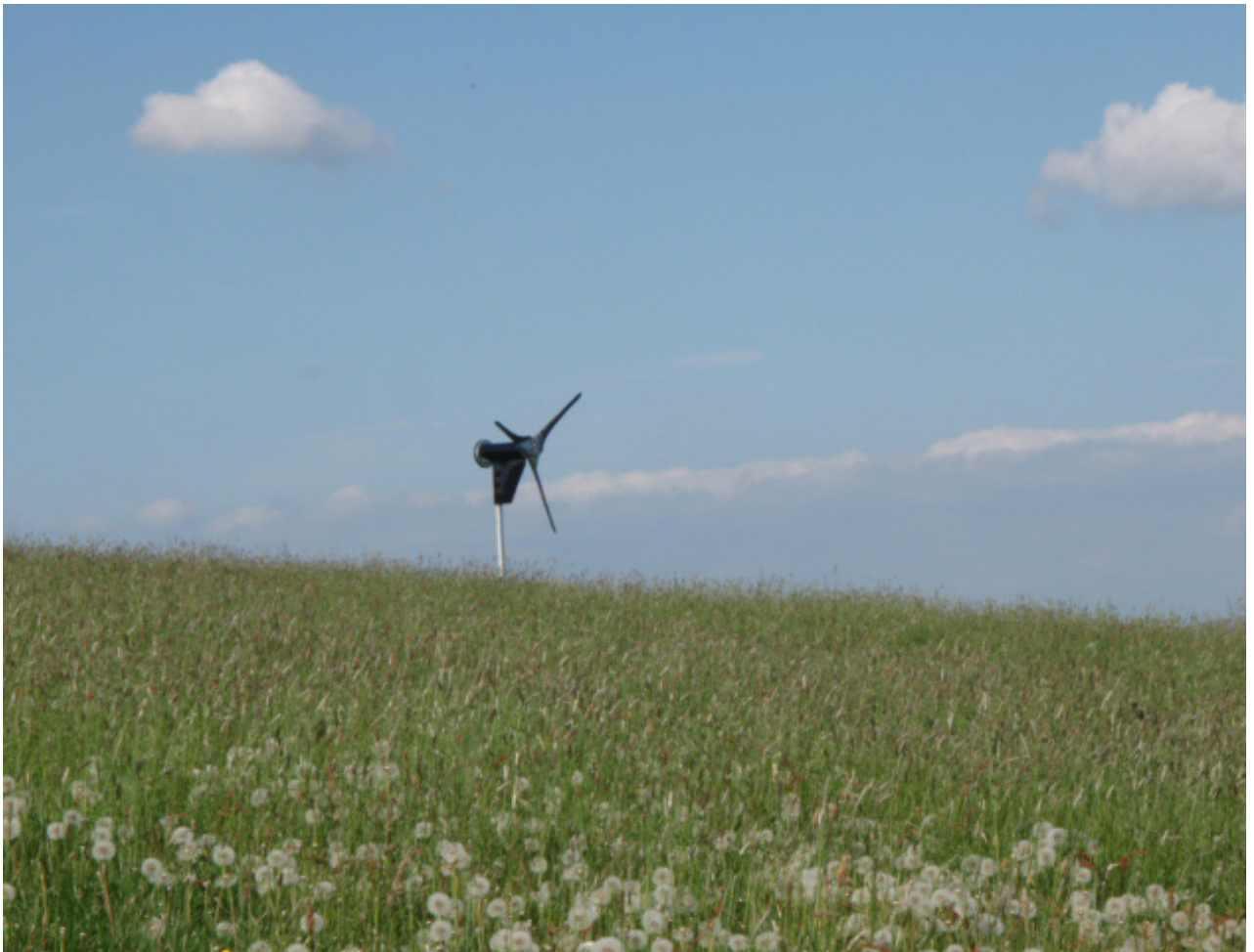
Figure 36. Example of a wind turbine breaking the ridgeline, demonstrating how skylineing can impact negatively on the natural beauty of the area if the guidance in figure 35 isn't achieved
