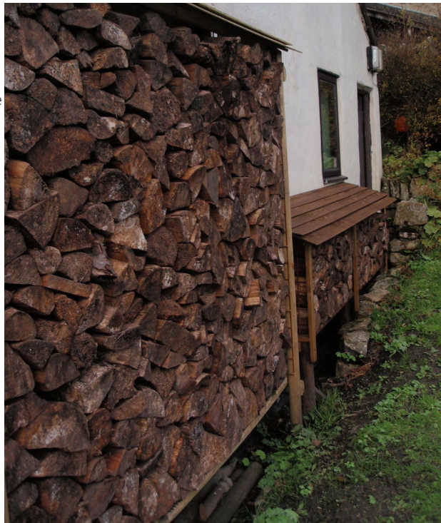
Figure 25. Wood fuel store for biomass stove
