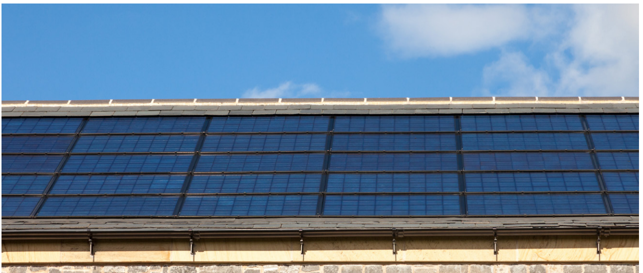
Figure 20. Flush fitted photovoltaic tiles
