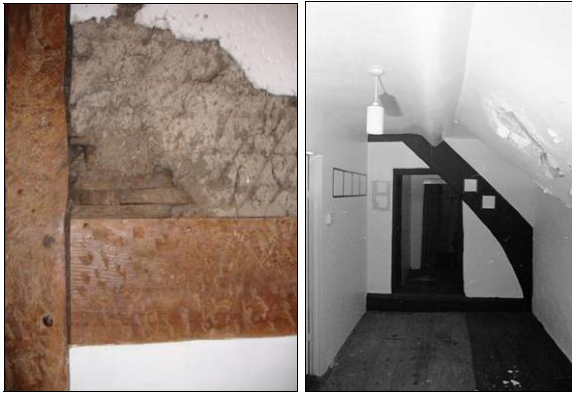
P6.28 Wattle and daub panel, Parsonage House
