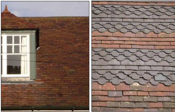
P6.40 Plain red clay tiles, North Church Street P6.41 Plain red and blue clay tiles and blue club clay tile roof covering, Rufford, Buxton Road
