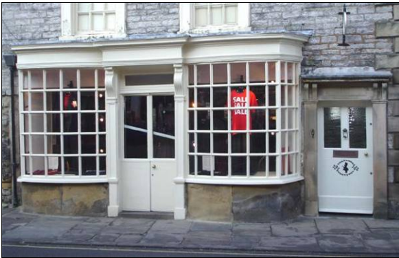
P6.7 Above: Gritstone stall-riser to traditional shop-front
