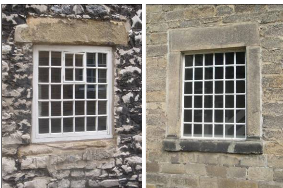
P6.46 Top Left: Timber sash window
