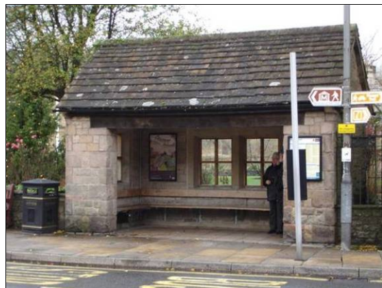
P6.89 Bus Shelter, Rutland Square
