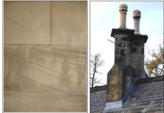
P6.11 Above Left: Ashlar P6.12 Above Right: Gritstone ashlar chimneystacks
