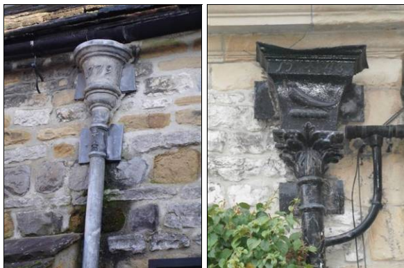
P6.42 & P6.43 Above: Examples of lead hopper-heads and downpipes
