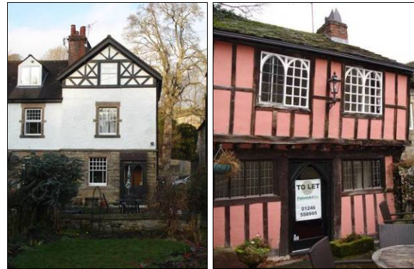
P6.31 Timber-framing, Lumford Cottages
