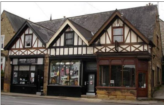
P6.30 Timber-framing to the upper storey of shops, Buxton Road
