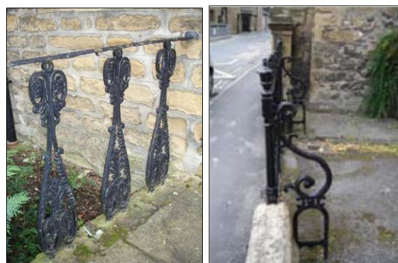
P6.59 Above Left: Railings, Rutland Terrace
