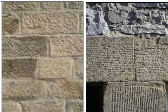
P6.8 Above Left: Quarter faced punched tooling P6.9 Above Right: Door Surrounds with narrow fluting and drafted margins
