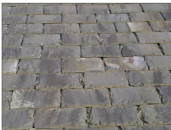
P6.39 Blue slate roof covering
