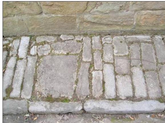
P6.70 Limestone setts and kerbs, Mill Street
