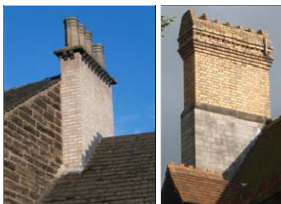
P6.23 Above Left: Gault brick chimneystack, North Church Street
