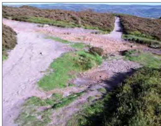
Extensive and increasing erosion at footpath crossroads close to cairn T2, October 2006. (Photograph: J. Hughes)
