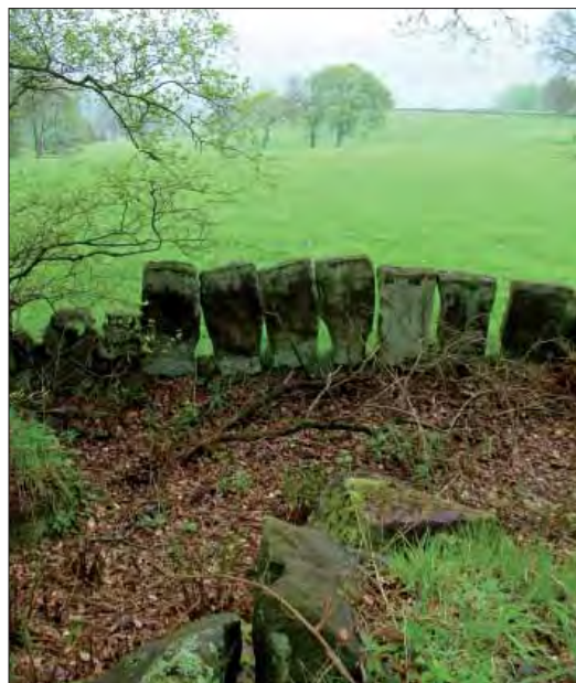
Gritstone slab wall on eastern edge of Sheepwalk Wood. (Photograph: S. McGuire)
