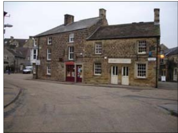
P7.64 Water Street looking north
