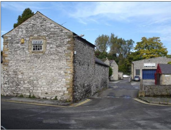
P7.40 View over Milford Bridge
