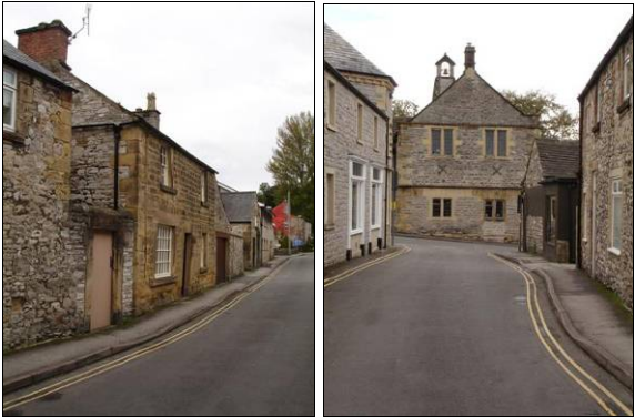
P7.116 Above Left: Buildings linked by high boundary walls
