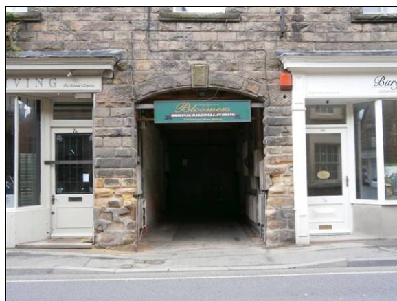
P7.84 Cart entry along Buxton Road
