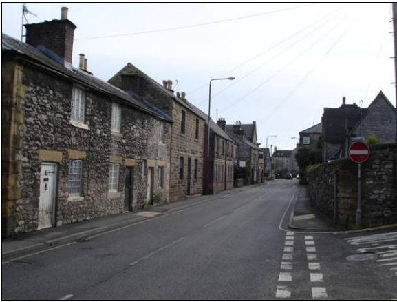
P7.86 View south down Buxton Road
