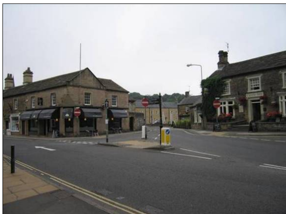
P7.52 East end of Bridge Street
