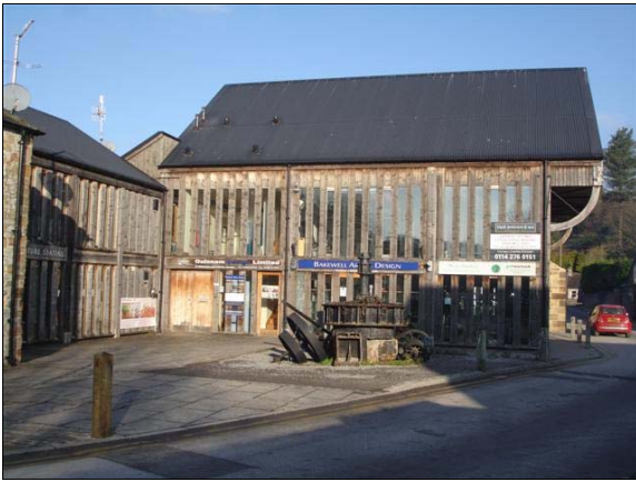
P7.28 Views terminated by a large building along Wood's Yard
