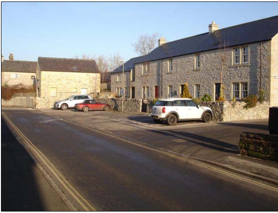
P7.63 View south along New Street
