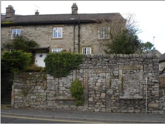
P7.140 The front elevation of a former building, part of a boundary along Monyash Road
