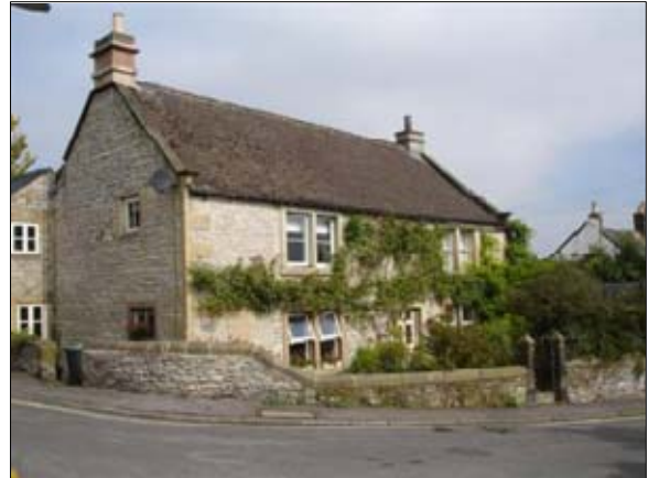
P7.156 Fellside, Stanedge Road
