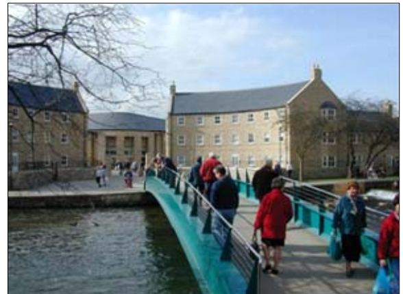
P7.30 Modern bridge leading to Riverside Crescent and the town-centre
