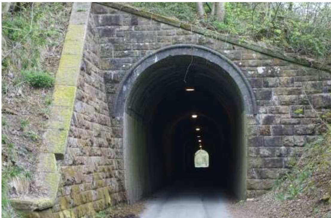
Figure 9.4 – Swainsley Tunnel carries an on-road section of the Manifold Track
