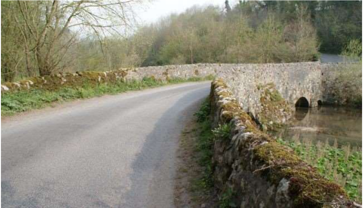
Figure 4.1 - Conksbury Lane and Bridge, part of the Youlgrave Quiet Lane Network
