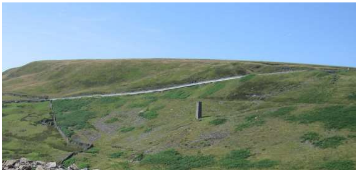
Figure 9.2 – A54 retaining wall and safety works, taken from Reave Edge Quarries
