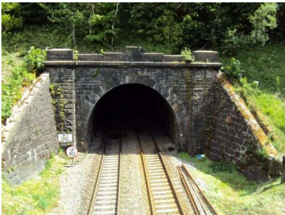
Figure 4.3 – Trolley Tunnel portal on the Hope Valley Line at Grindleford
