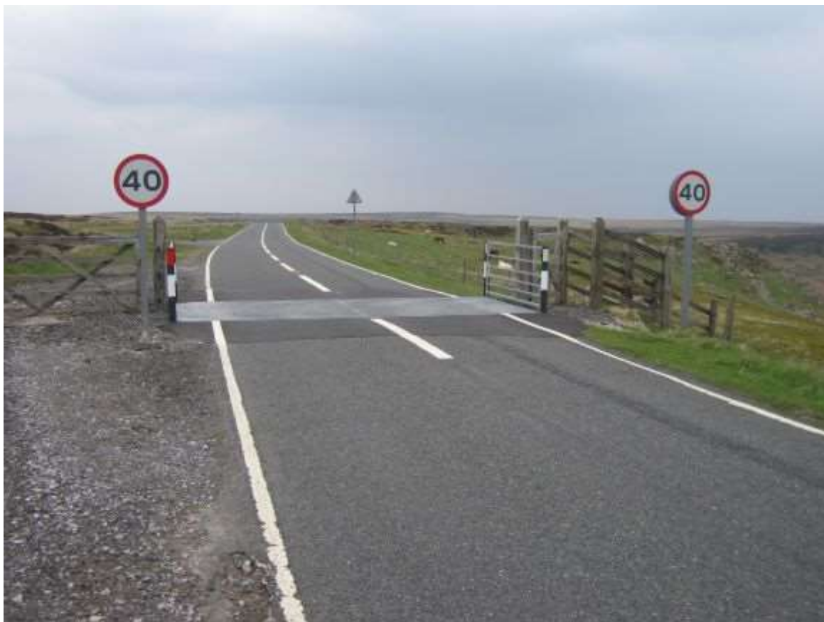
Figure 6.6 - Entrance to the North Lees / Stanage Traffic Management Scheme
