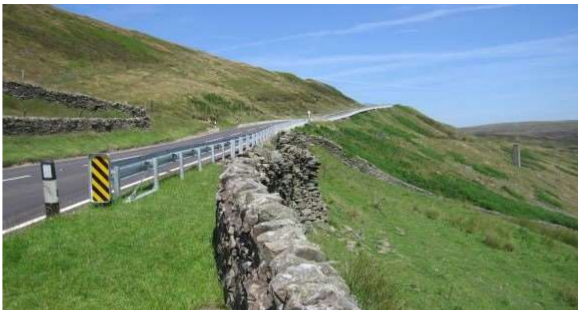
Figure 9.1 – A54 retaining wall and safety works
