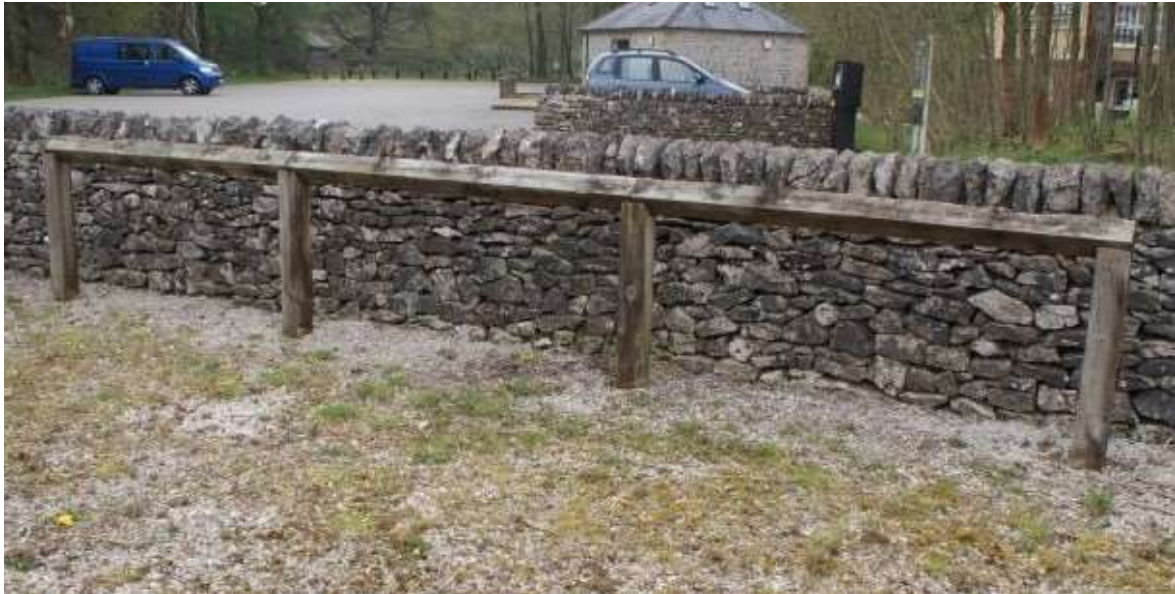
Figure 10.8 - Hitching rail at Hartington Station Car Park
