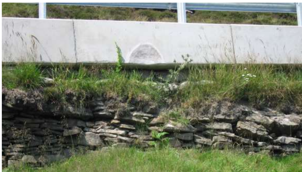
Figure 9.3 – A54 retaining wall and safety works, incorporating re-walling and revegetation
