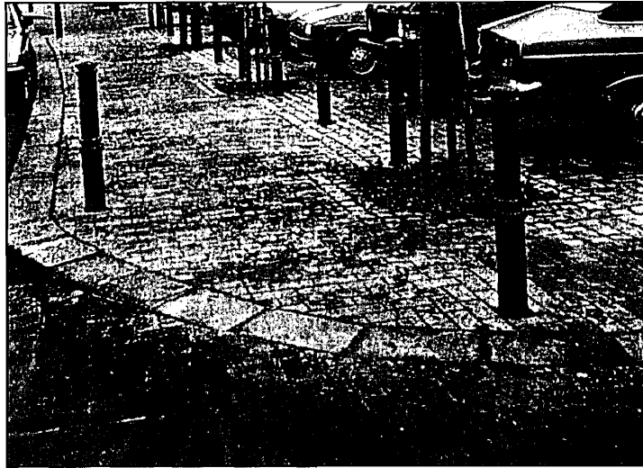
Concrete block paving with stone curbs and setts. Steel bollards of traditional design.
