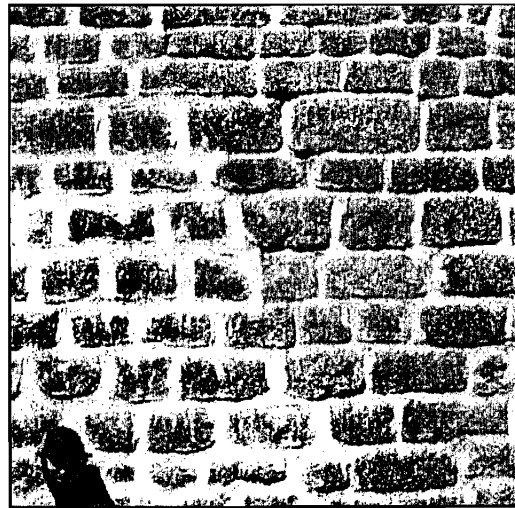
Bad pointing . . . joints too thick.
