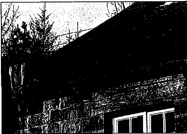
Timber guttering on stone corbels.
