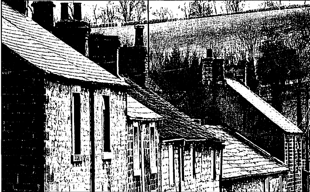
Flush verges; clipped eaves.
