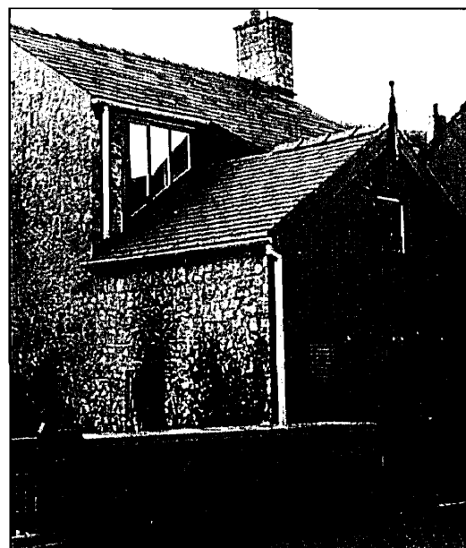
Conversion of joiner's shop to dwelling. Tideswell.
