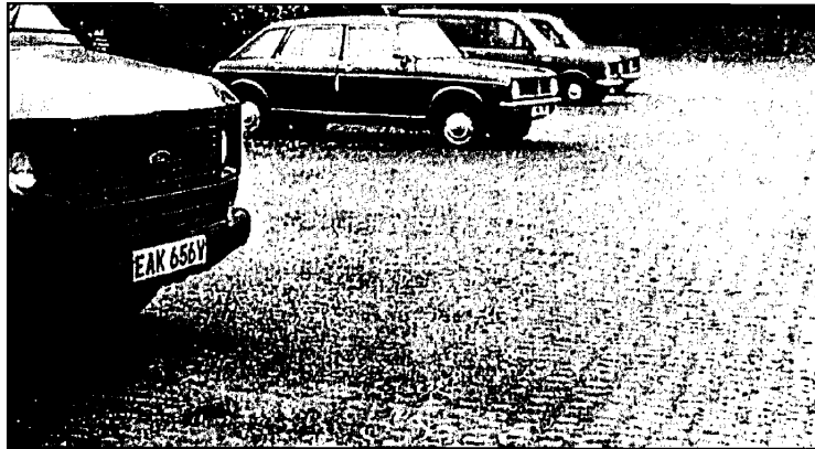
Car park surfaced with concrete/grass grid.
