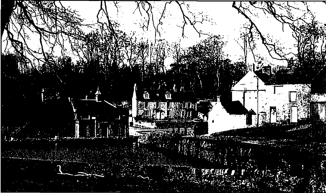
Open village with buildings well-spread allowing views of Monyash surrounding countryside: a feeling of spaciousness.
