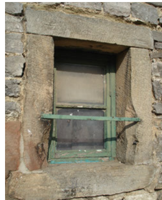
A like-for-like replacement of an historic window, including stonework repairs and new ironwork, based on evidence from the existing openings. (© Bench Architects)
