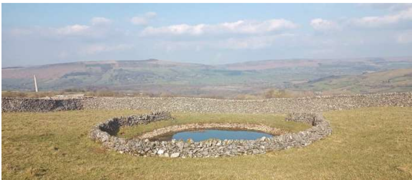
5 FiPL- Paradise Farm pond restoration- finished scheme
