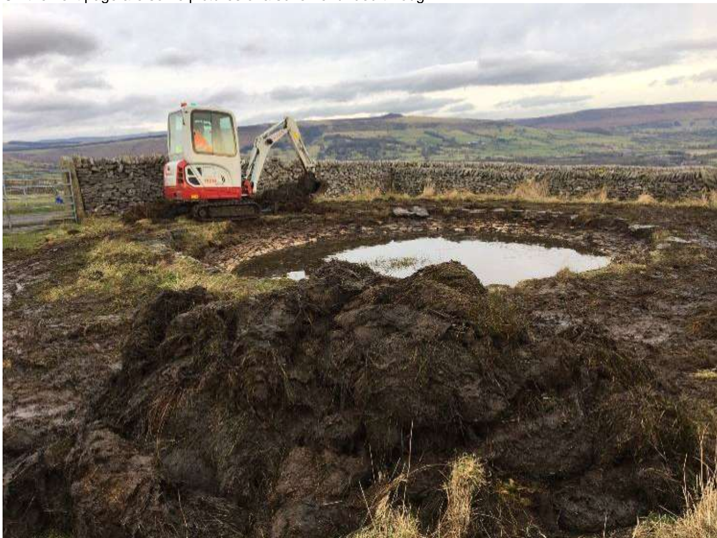
4 FiPL- Paradise Farm Pond restoration - work in progress
