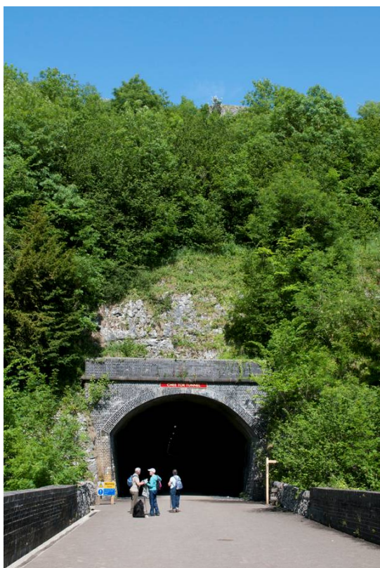
Southern portal of Chee Tor Tunnel
