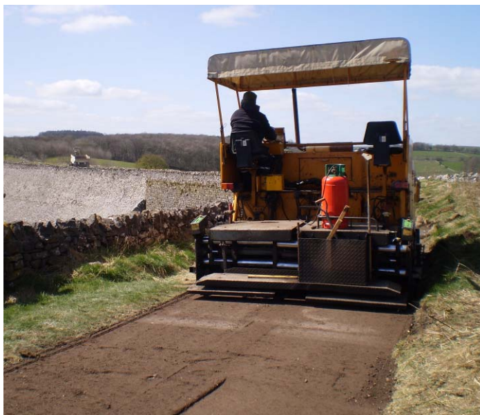
Re-surfacing on High Peak Trail
