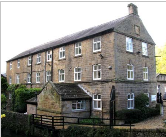
P10.1 Lumford Mill former workshop, now included within the Conservation Area boundary
