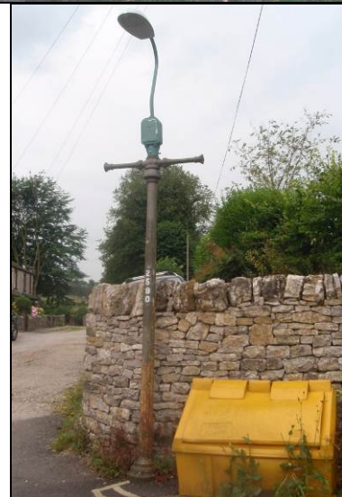
P11.6 Streetlights positioned next to each other (top) and traditional lamp posts (top-right and bottom) in poor condition, with modern lamps
