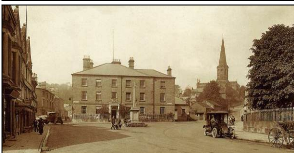
P11.3 Historic photographs showing the original railings to Bath Gardens; their reinstatement would be a positive enhancement
