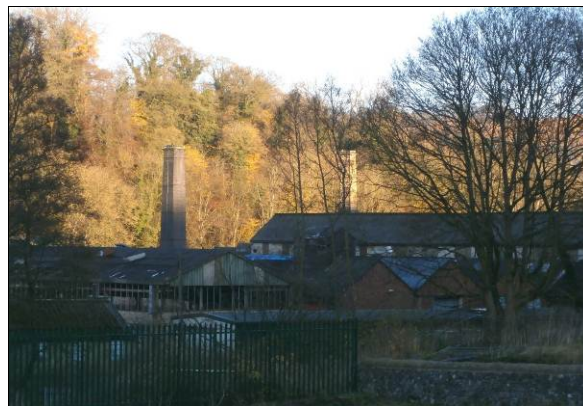
P9.5 The chimneys at Lumford Mill
