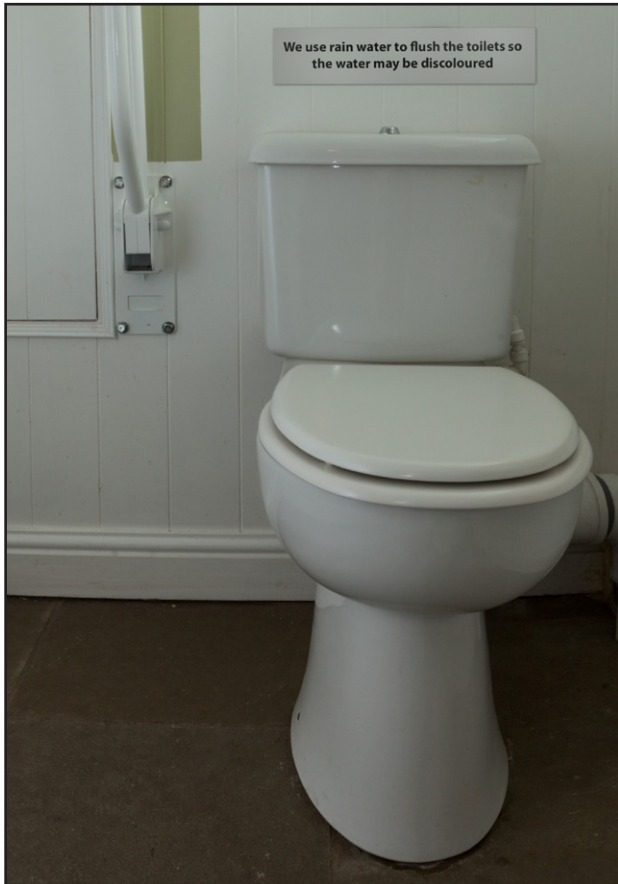
Figure 2.11 Rainwater harvesting for toilet flushing
