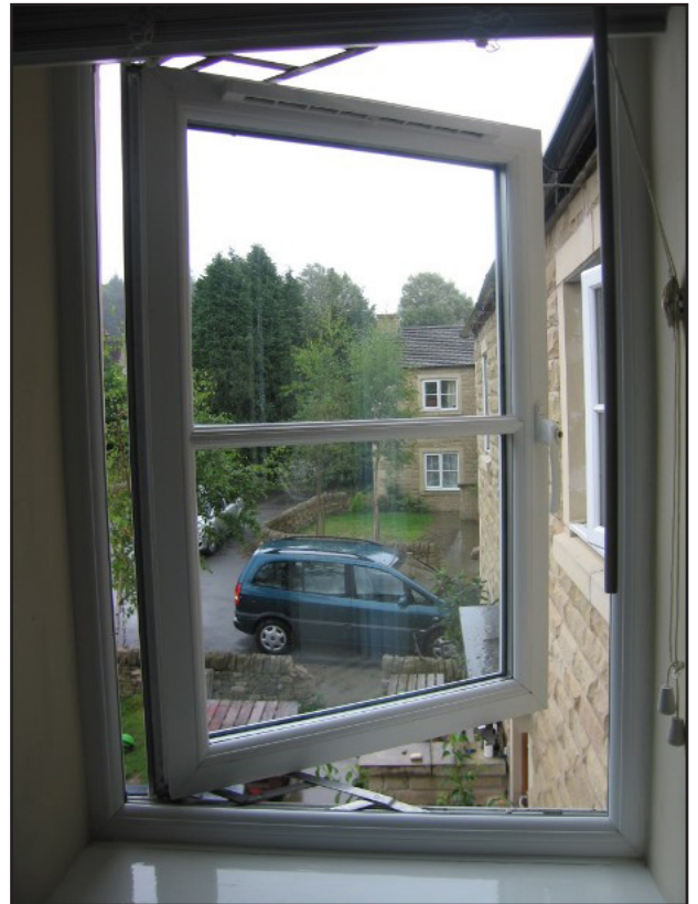
Figure 5.4 Double glazed window with low emissivity glass.
