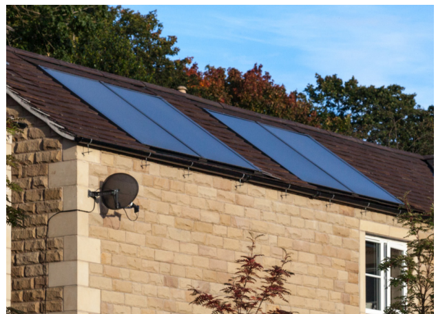
Figure 5.5 Solar panels on the roofs.
