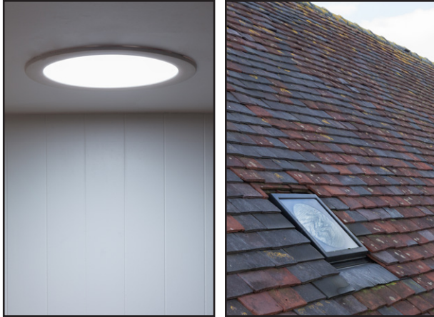
Figure 2.7 Sun Pipe – minimal impact on Grade II listed building
