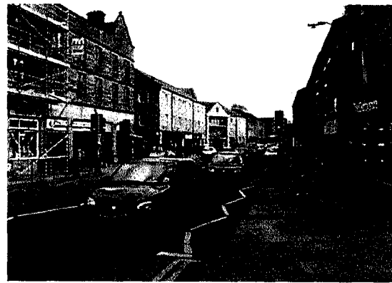
Build out the pavement on either side of the crossing
