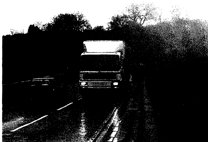
Conditions on the Bridge are hazardous for pedestrians
