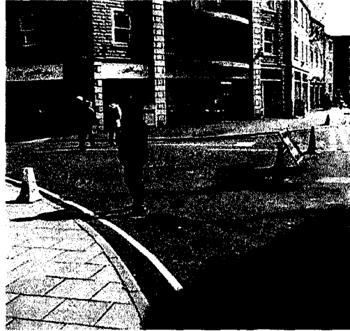
The tactile paving to cross this junction is just visible on the far left of this picture - considerably away from the desire line
