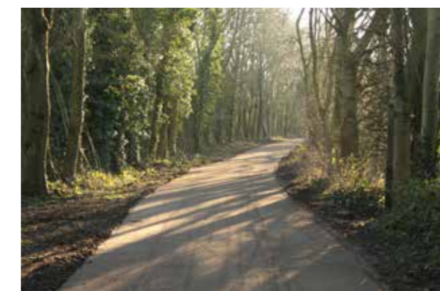
Tissington Trail after improvement works
