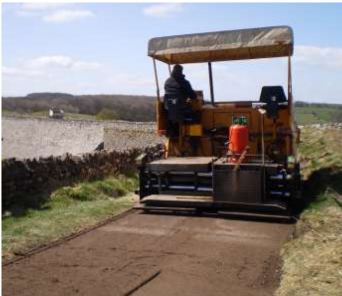
Re-surfacing on High Peak Trail
