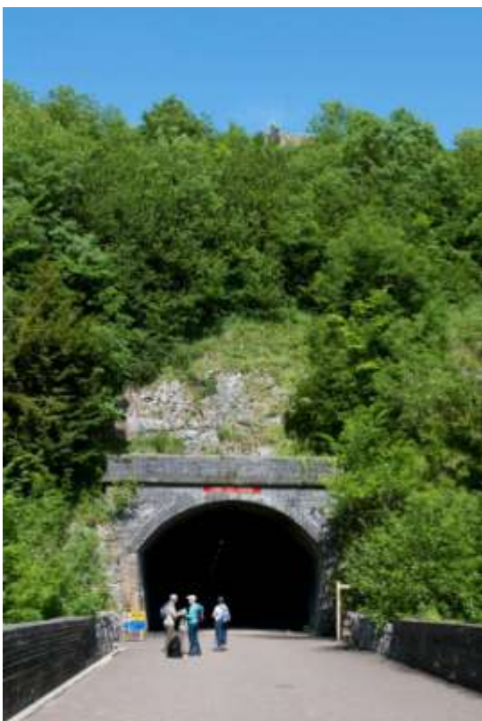
Southern portal of Chee Tor Tunnel
