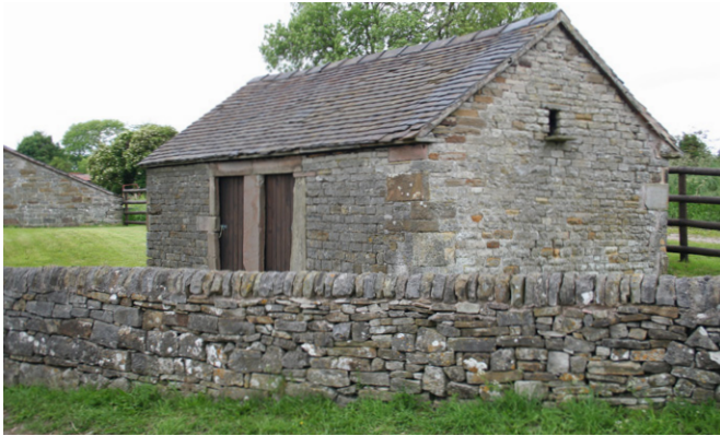
This small cow house stands in a small paddock within a village rather than being part of a formal farmstead. Note the pophole in the gable end for hens, which would access the henloft via a moveable ladder. Photo © Jen Deadman
