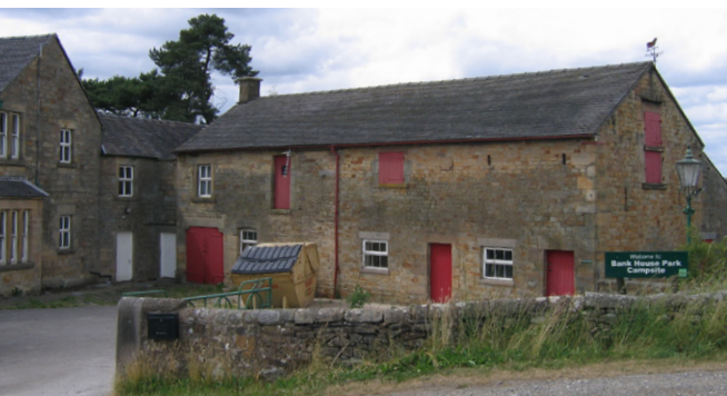
A combination barn with an integral cartshed to the left. Photo © Jen Deadman
