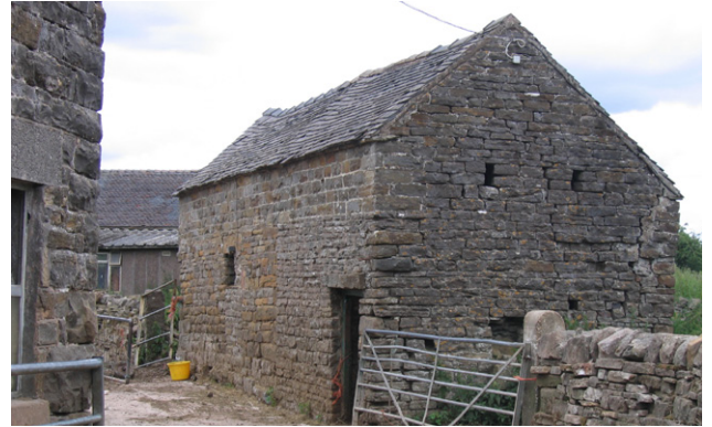
A small-scale animal house, the larger stone blocks indicating the raising and extension of an earlier stone rubble building. Photo © Jen Deadman
