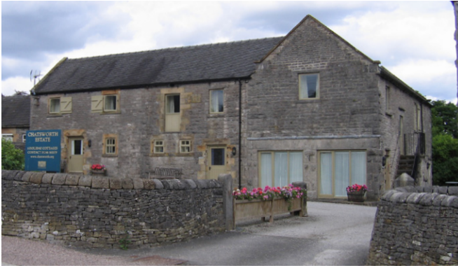
A combination barn remodelled into its present form in the late 19th century, and now houses offices. The steps to the right provide access to a granary sited above a cartshed. To the left is a cowhouse and (far left, marked by its taller door) a stable. Above is a pitching door to the loft for hay and the corn crop. Photo © Jen Deadman
