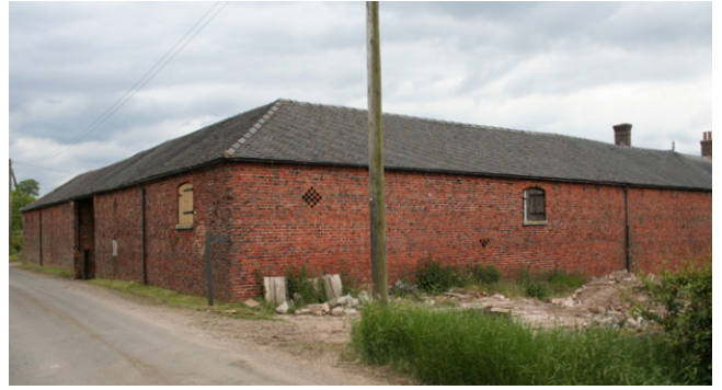
In contrast to the usual stone farm buildings this brick-built regular U-plan farmstead is more typical of lowland areas of Staffordshire. Photo © Jen Deadman
