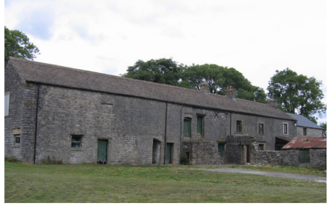
Linear farmsteads often developed over the 18th and 19th centuries into substantial ranges – ground-floor stabling and cattle housing and first-floor granaries (marked by the steps to right), hay loft and storage for the corn crop. Photo © Jen Deadman
