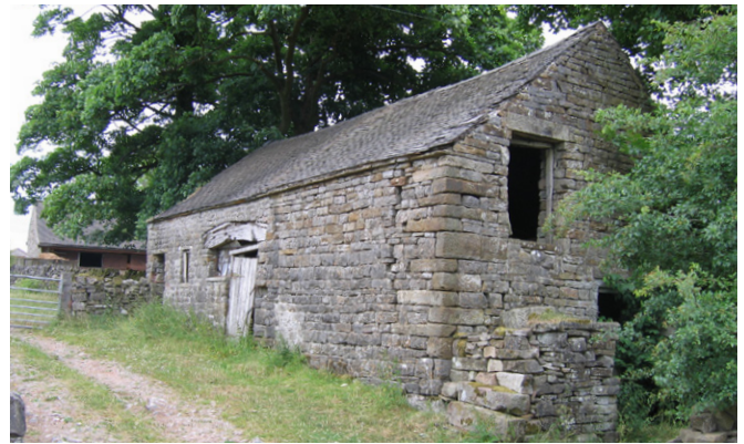
Combination barn with lofted cattle housing accessed from the gable end. The central threshing bay has a stable beyond. This form of barn was more common before the rebuilding with large storeyed barns in the 19th century. The lintel over the threshing door is a possible remnant of a timber-framed building, these having been largely swept away by stone buildings by the 19th century. Photo © Jen Deadman
